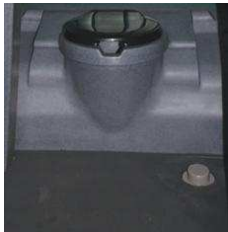
Foot pump flush
